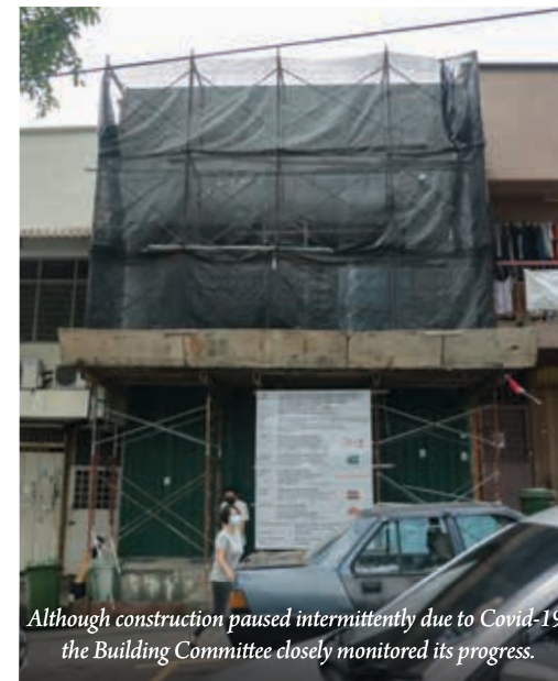
Level 1 of the new Centre will feature the Library & Resource Centre. Its versatile built-up can be repurposed for various uses and programmes.
