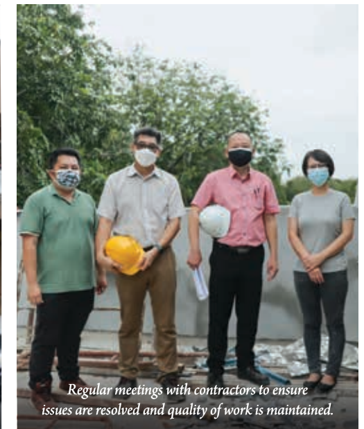
Although construction paused intermittently due to Covid-19, the Building Committee closely monitored its progress.
