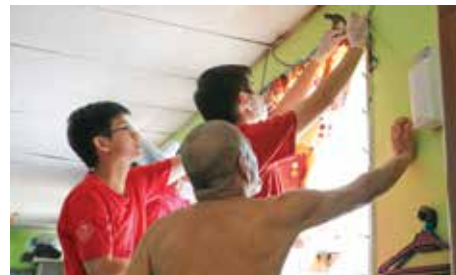
Helping to fix and repair facilities at the home.
